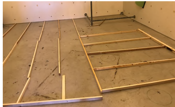
Spacers laid out before mounting of Acupanel
